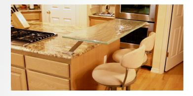
your first bracket. Make sure that when you fasten the bracket that you check for level in all directions. The bracket should be straight up and down and be level across the top flange as well as down the top flange. This will give the bet possible support result to your countertop.
